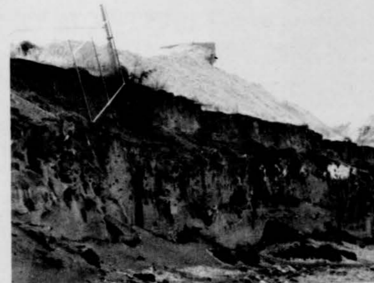
RC&D funding was received to help stabilize streambank erosion at the Port of Morrow.
