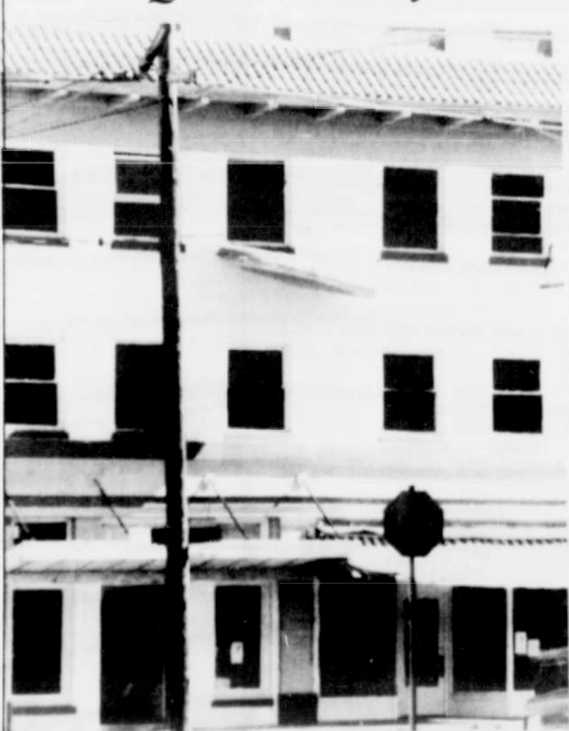
Someone at the Heppner Hotel project was getting prepared last week for "the big one" by putting a rubber boat out the hotel window.
