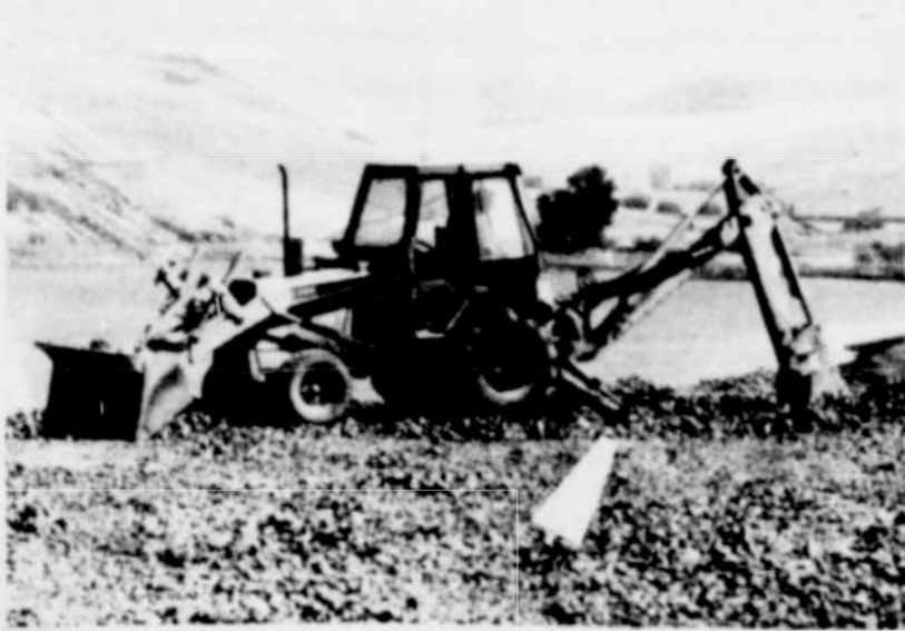
Work has begun on the Willow Creek Park Project.
