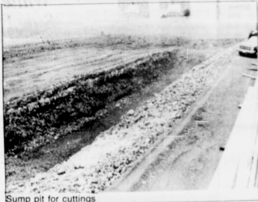
Sump pit for cuttings
