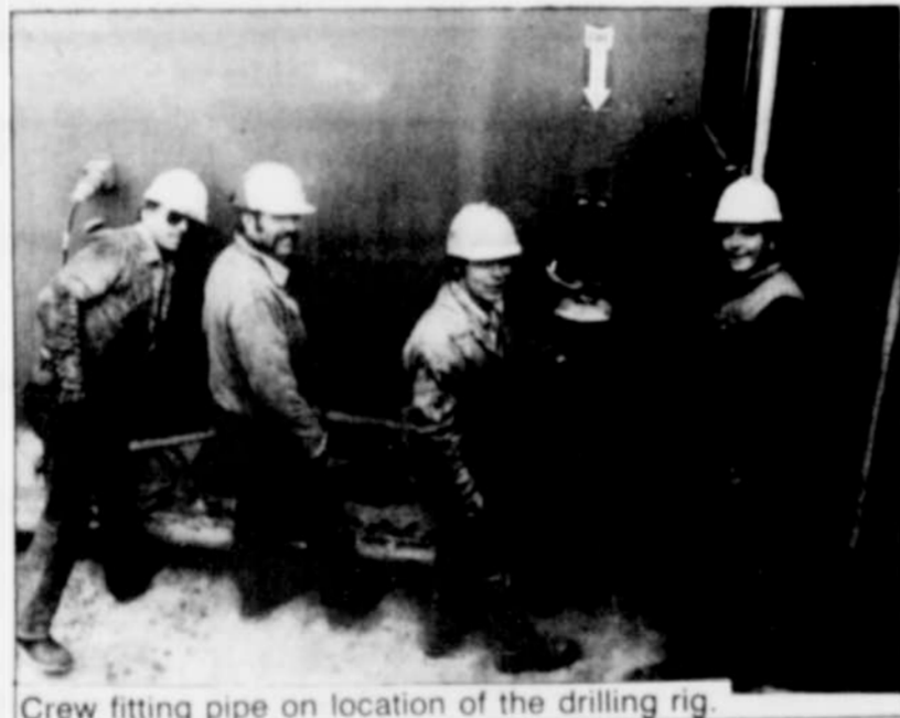
Crew fitting pipe on location of the drilling rig.
