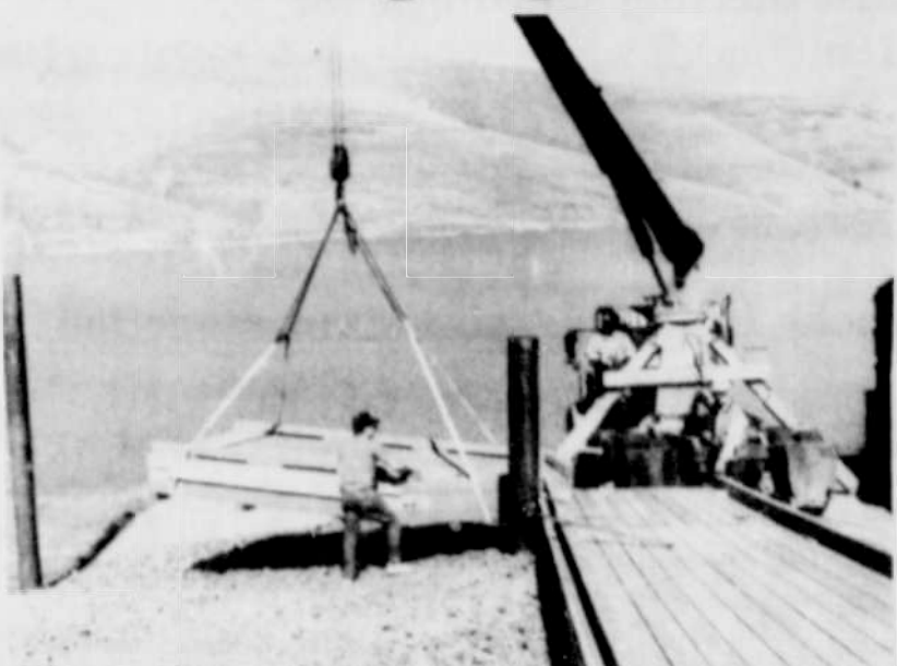
These men are installing the new docks at the Willow Creek Lake on Tuesday. They were in place by the end of the day.
