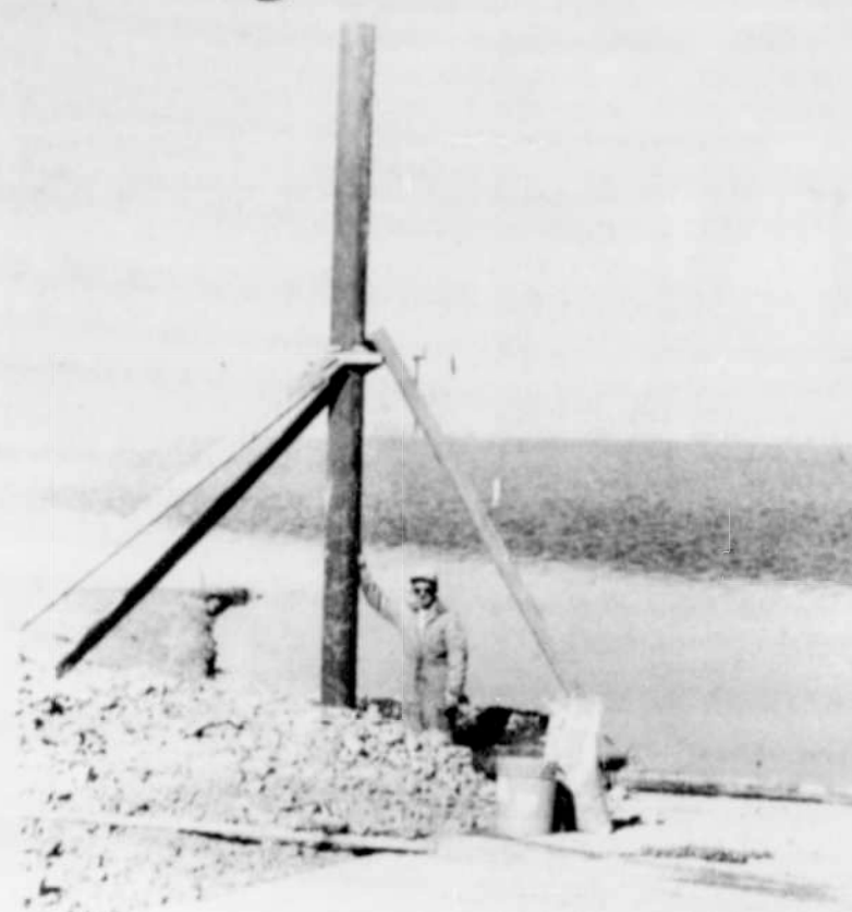
Bert Corbin is standing beside one of the pilings being put in place this week at the Willow Creek Dam boat ramp. Bert, along with Miller and Son Welding are doing the work for the Willow Creek Park District. The docks will not be put into place probably until next fall because of the level of the water.
