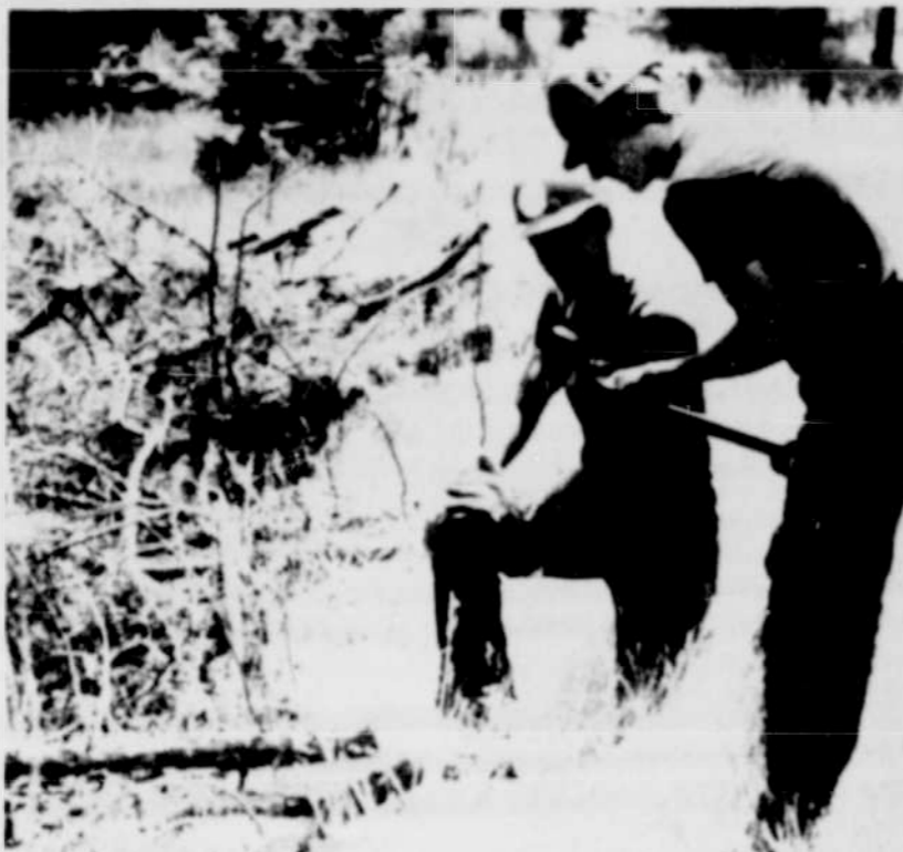
Craig Angell (left) and John Steagall drive stakes to secure junipers to streambank.
