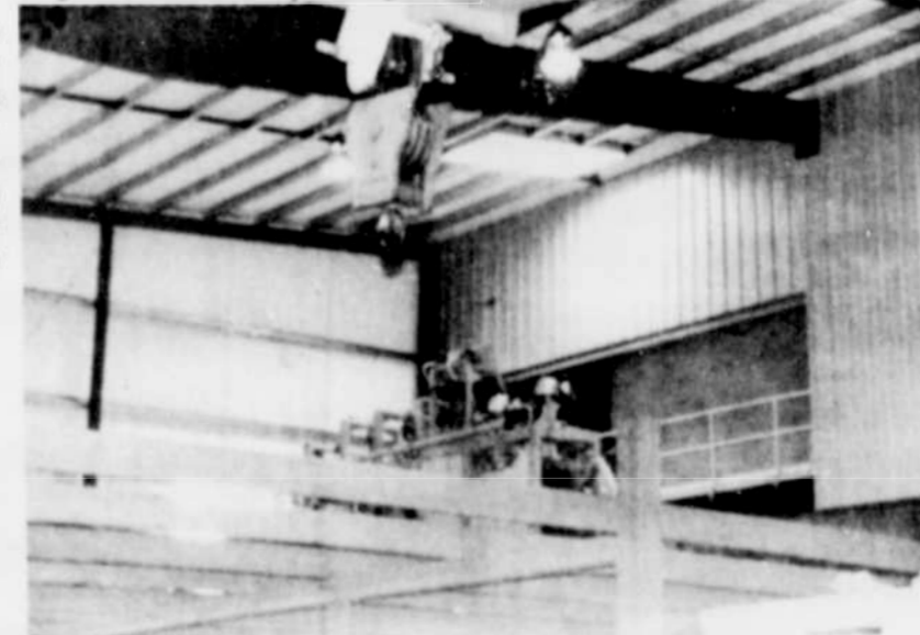
Crane and first of saws installed at stud mill.
