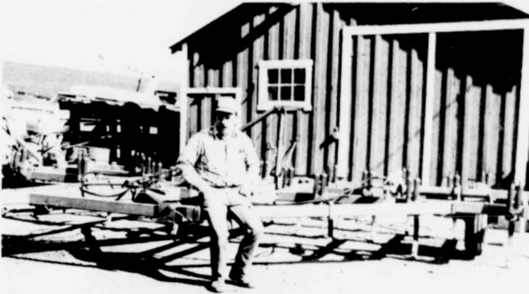
Ken Nelson sits on chisel plow which he uses instead of a moldboard plow to work the sandy soil on his farm near Lexington. The plow helps to conserve moisture and prevent soil erosion.
