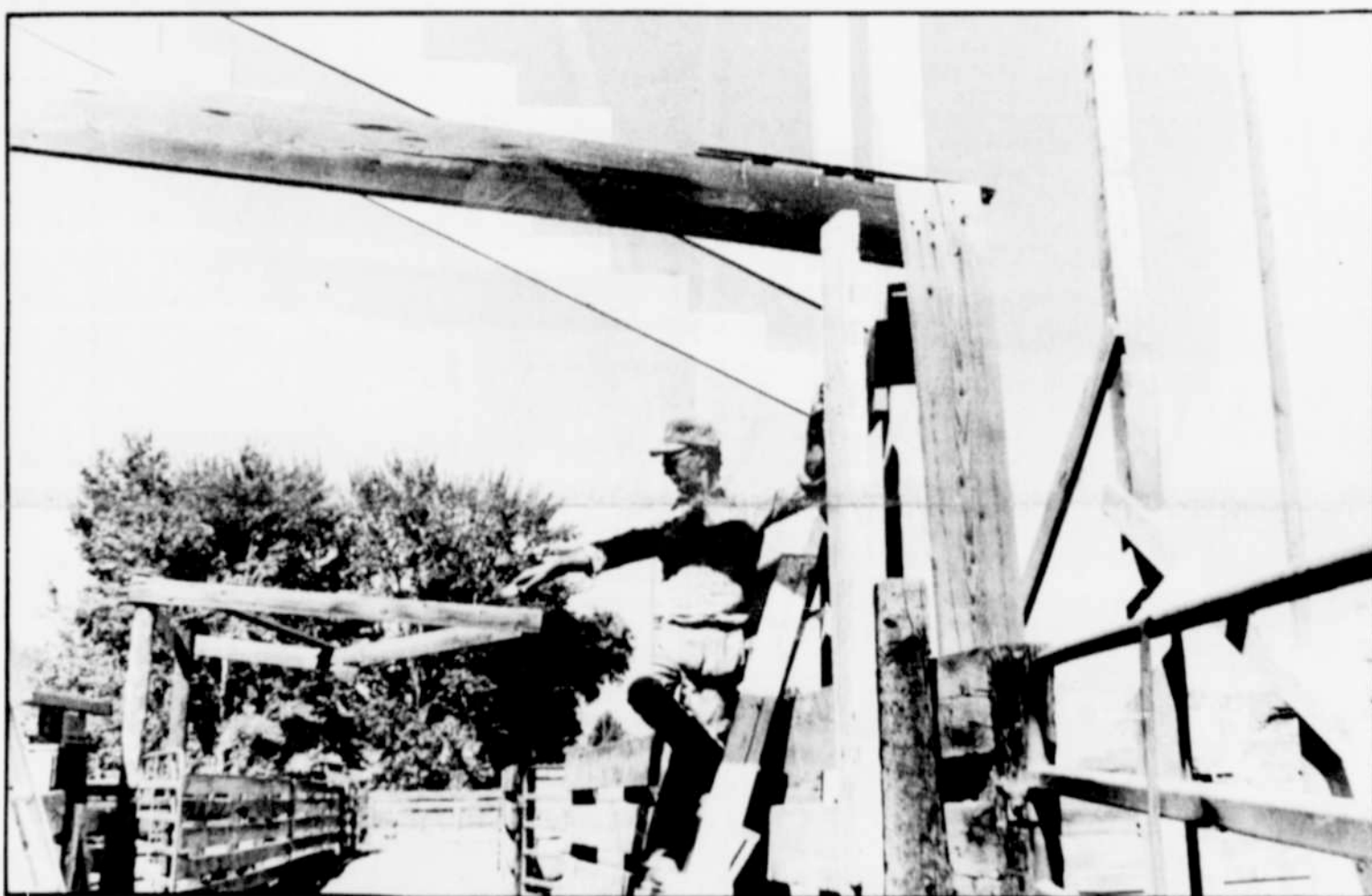
Building an escape
