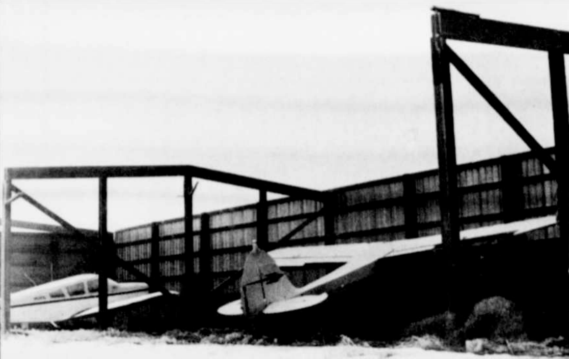
Hangar at Lexington airport
