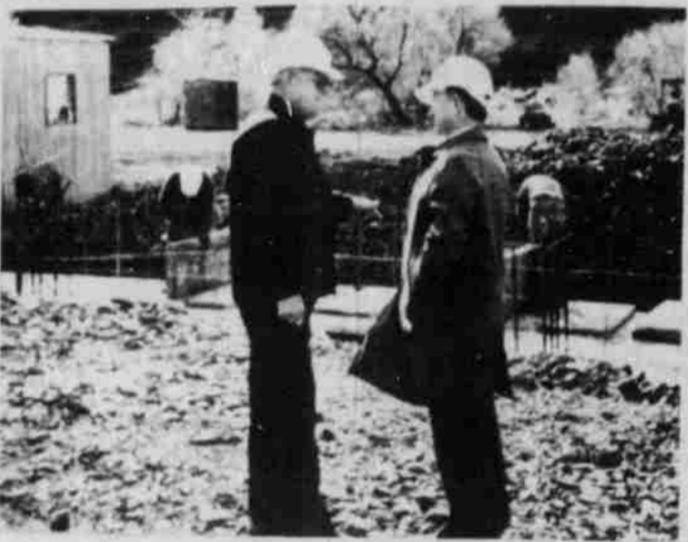
Harry Kennison (left), general manager at Kinzua Corp. talks with Bill Braun, the engineer who drew the plans for the co-generation plant.
