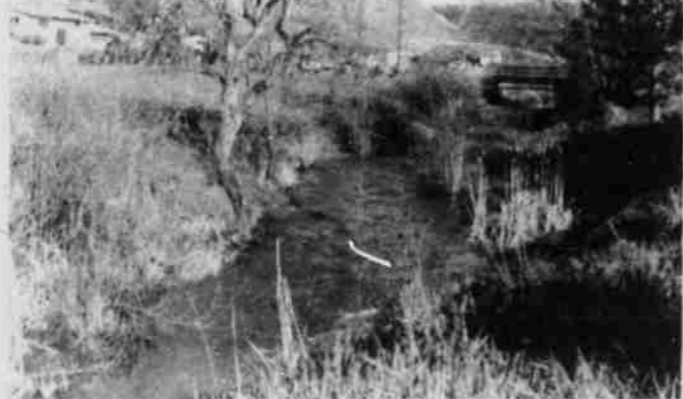
Grass and weeds are overgrown along the banks of the creek.
