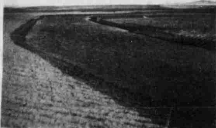
Level terraces such as this have worked effectively to reduce erosion and runoff. Terraces are designed to store 1.3 inches of runoff per acre.
