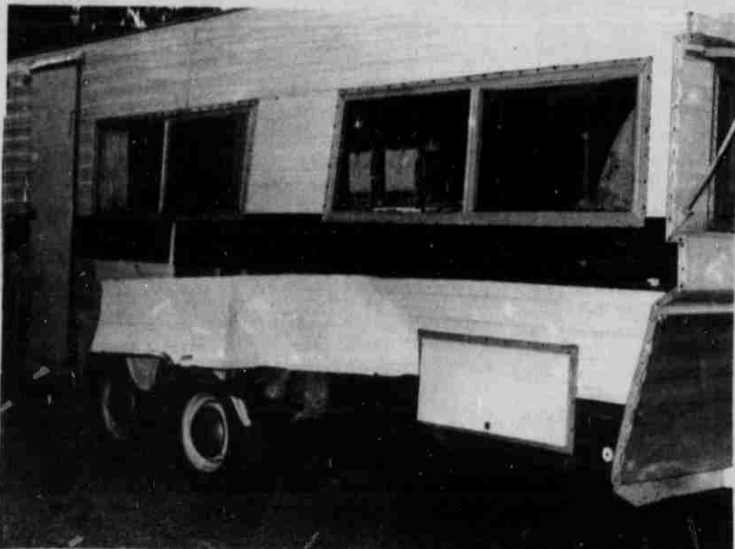
Propane explosion caused extensive damage to trailer at Cutsforth Park Friday night.
