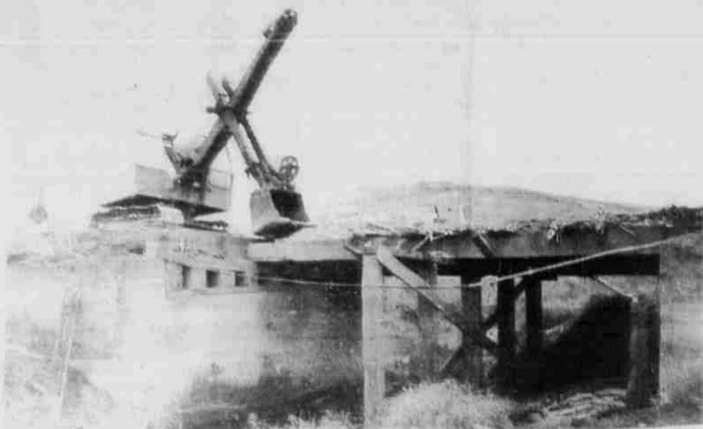
An old Lexington bridge was removed Monday
