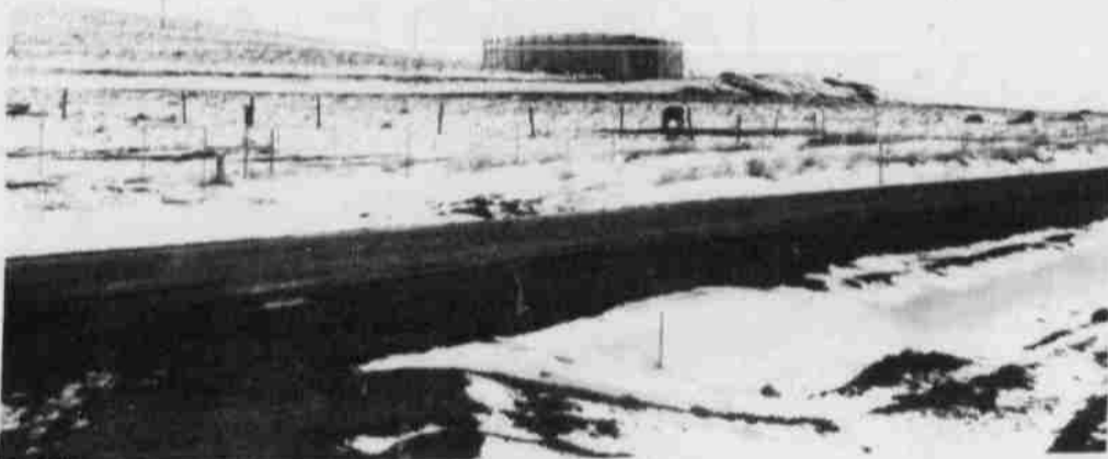
Heppner's new water tank is under construction
