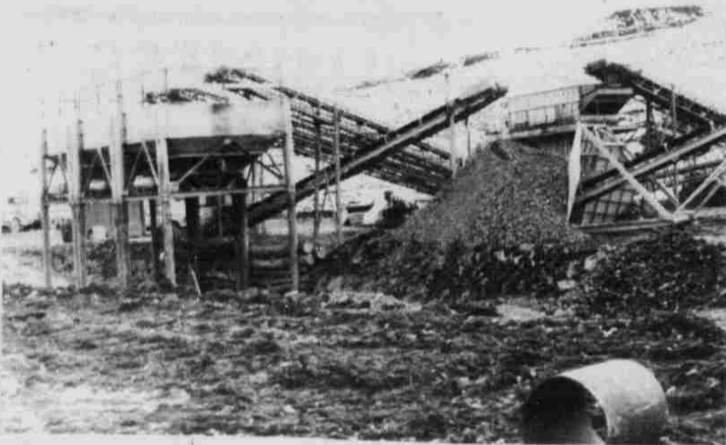
Two shifts of workers operate the aggregate crusher
