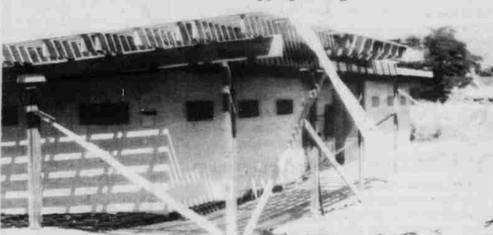
Construction underway at Heppner swimming pool
