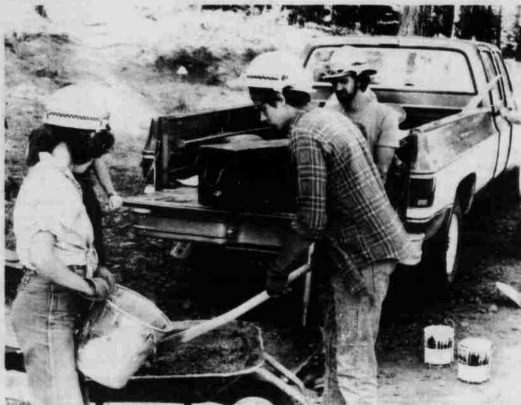
John Brennan prepares concrete for fire ring installation.
