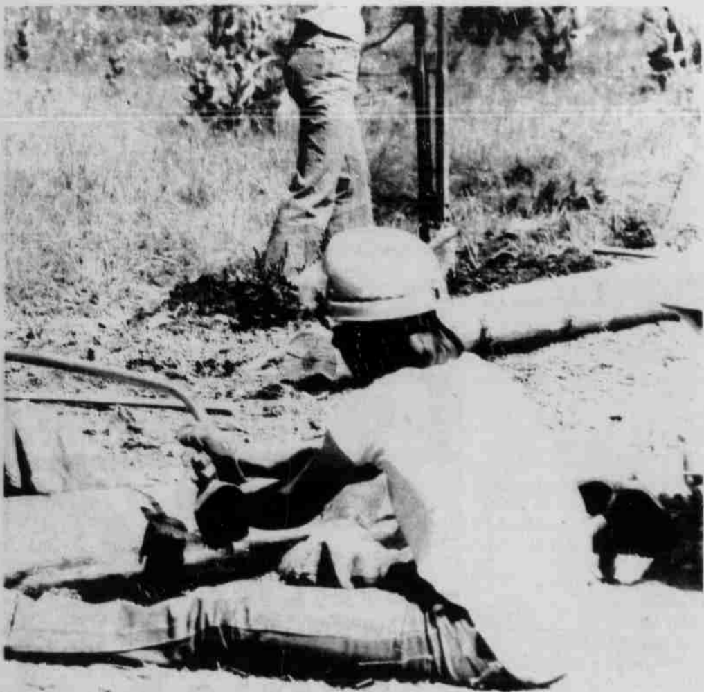
Casey Weisman saws logs for traffic barrier posts at Bull Prairie Lake.
