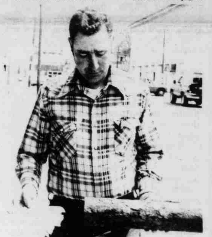
Clifford Green ponders about the holes in the pipe of the city water system.
