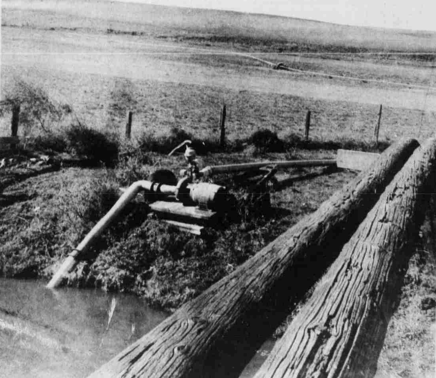
Irrigation pumps like this one taking water out of Willow Creek have been the center of controversy this past week.
