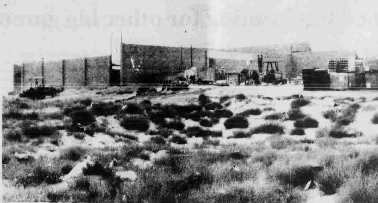
New School The new Sam Boardman Elementary School is rising on the Boardman horizon. Located near a new housing subdivision, the school is one of new structures being built for north end students. The new Columbia Jr. High will be located between Boardman and Irrigon.
