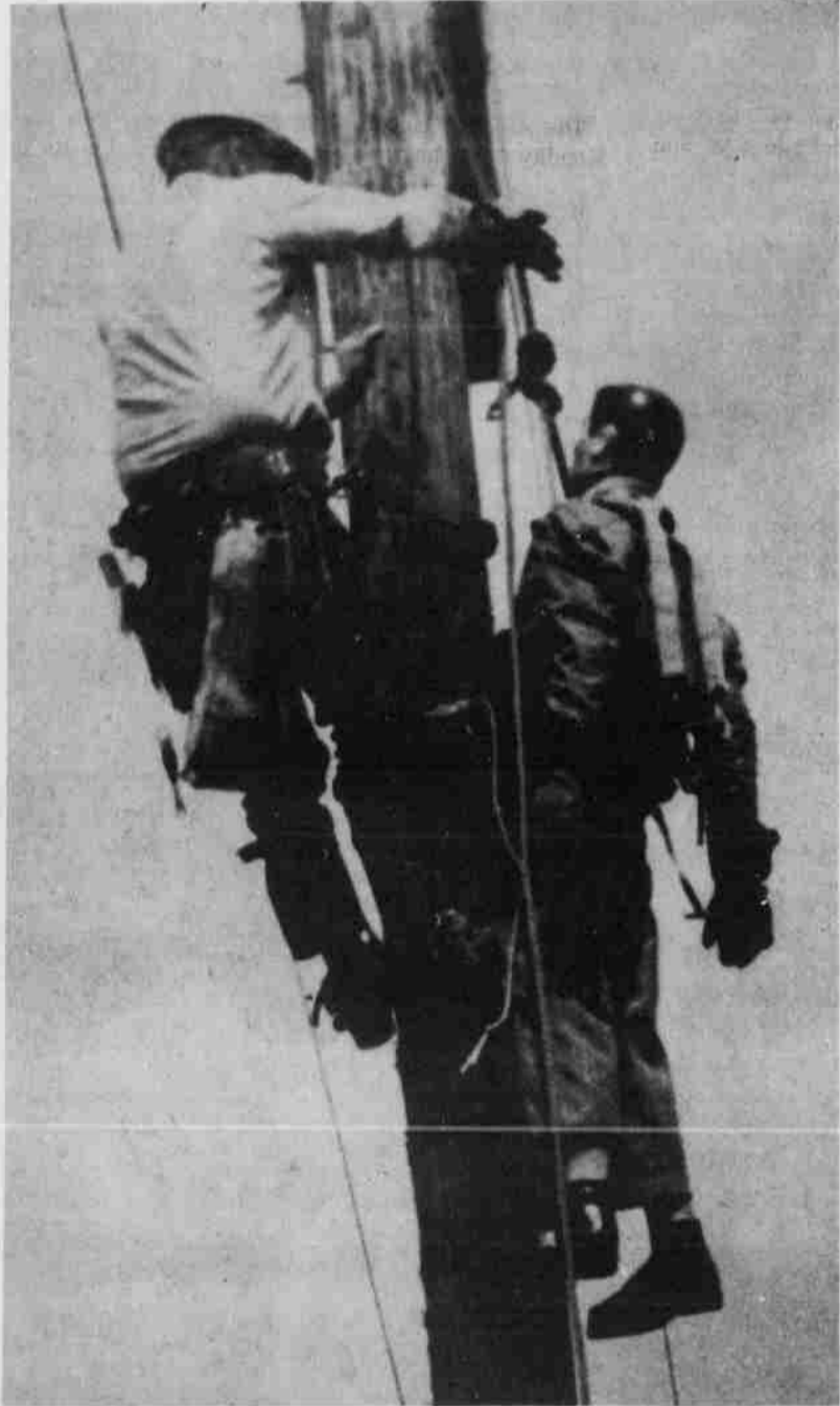
Columbia Basin Electric Cooperative employee Doyle Key tries his hand at rescuing an "injured co-worker from atop a power pole. The "co-worker" in this case is a "dummy".
