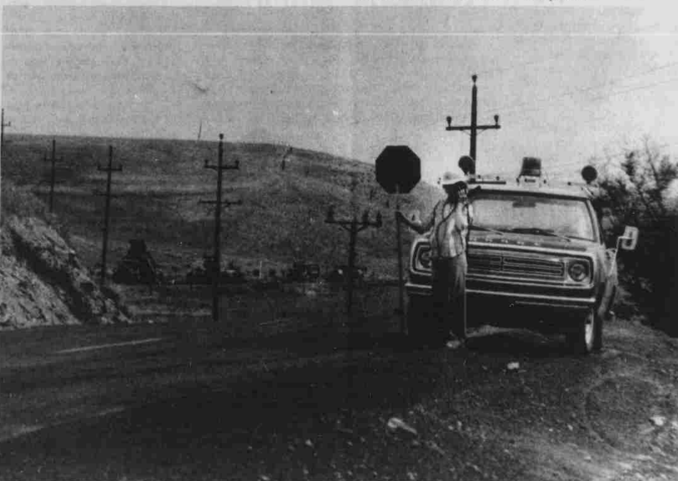
Laying it down
