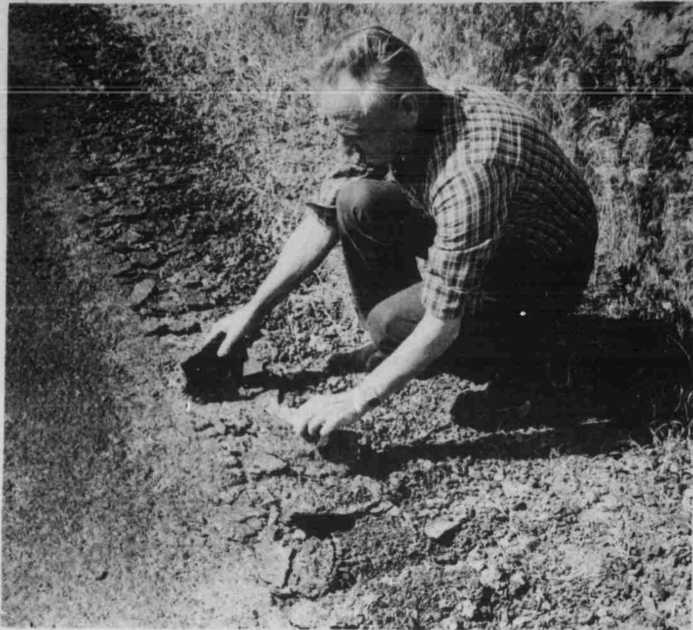
County Roadmaster Doc Sherer shows broken pavement along Ione-Boardman Road caused by a Caterpillar-type farm tractor. The clefted tractor tore up the edge of the county road for more than a mile. Most of the route it traveled was along empty summer fallow land, on which it could have moved without causing damage. Sherer figures it will cost more than $600 to repair the road. Similar damage is common on county roads, he said.
