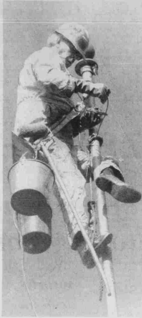
Bill Hinrichs shows how one leg wrapped around the pole secures his position as a steeplejack. The pole in the picture sits in front of the Morrow County Courthouse.
