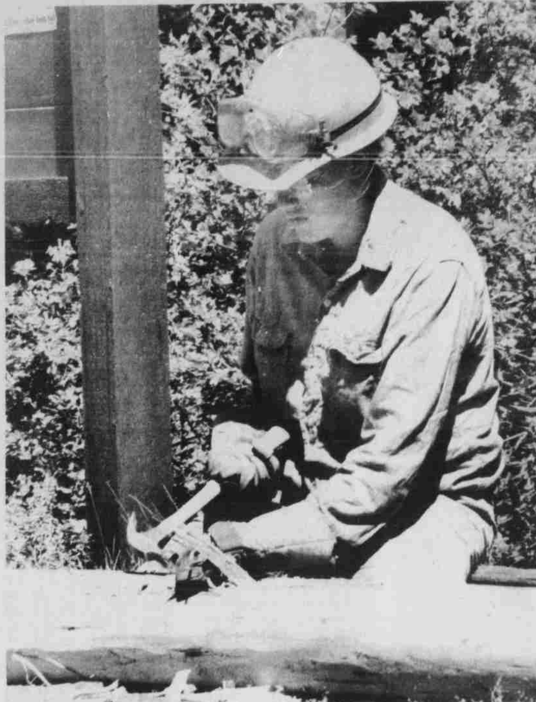
Working with the hands in constructing a pole fence starts in the forest with the cutting of the trees, then peeling of the poles and chiseling notches.
