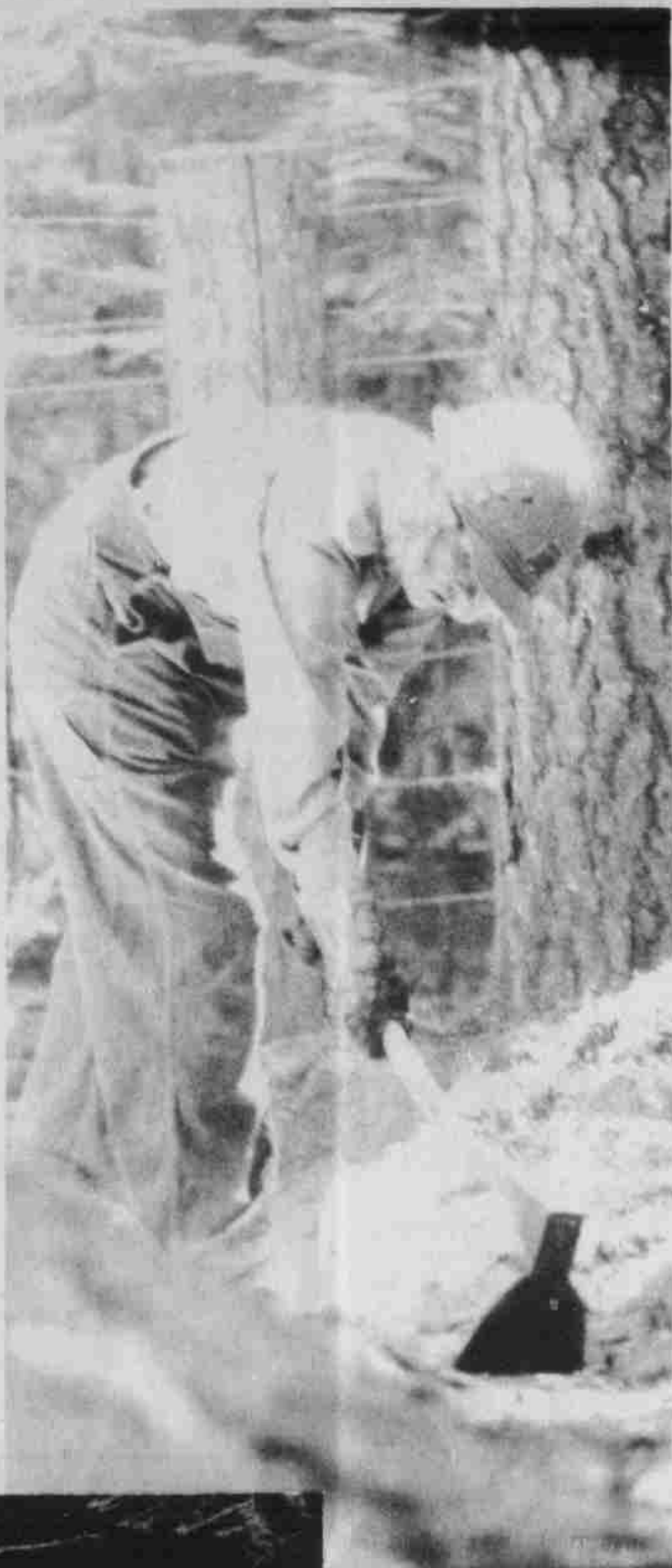
Working with the hands in constructing a pole fence starts in the forest with the cutting of the trees, then peeling of the poles and chiseling notches.
