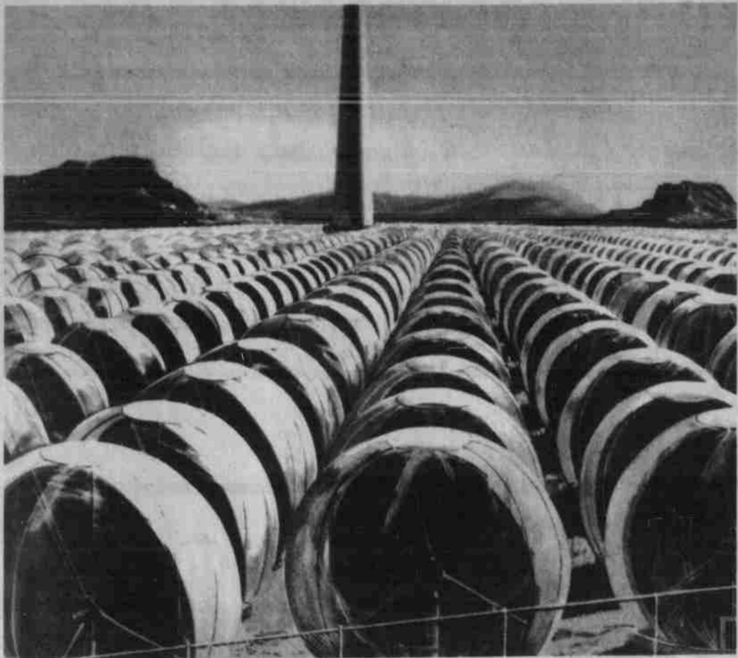
Field of heliostats could produce energy equivalent to a 10 megawatt power plant.
