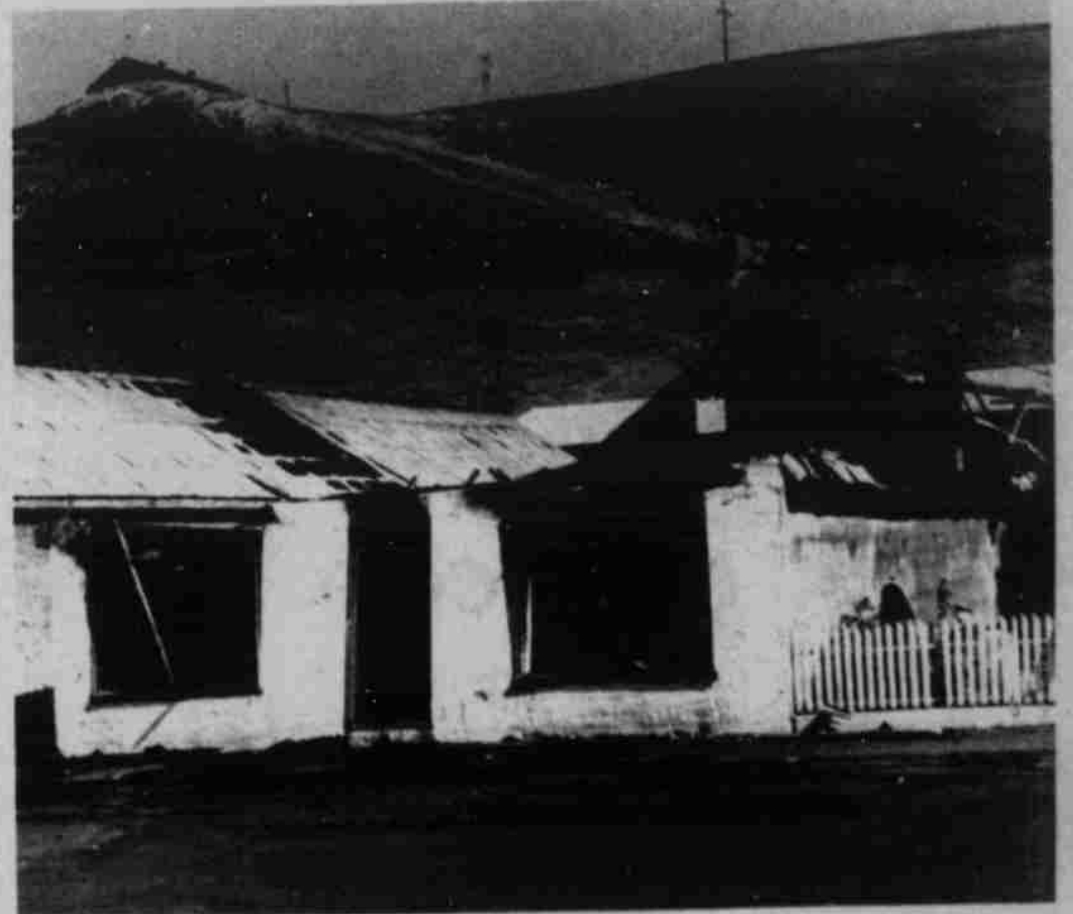
An early morning fire in lone Friday gutted the Art Stefani building and jumped to adjacent roof.
