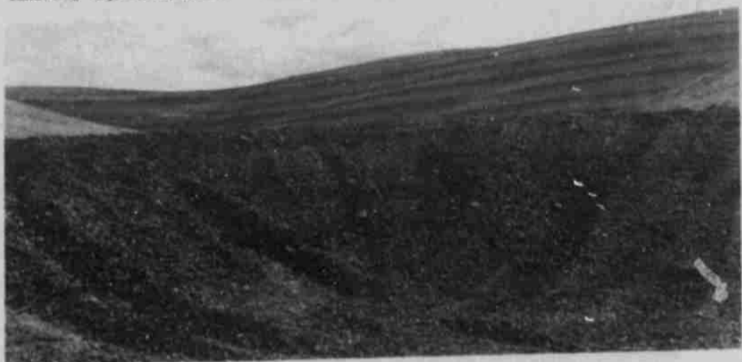
A silt dam, foreground, and diversion ditches, background, south of Heppner.
