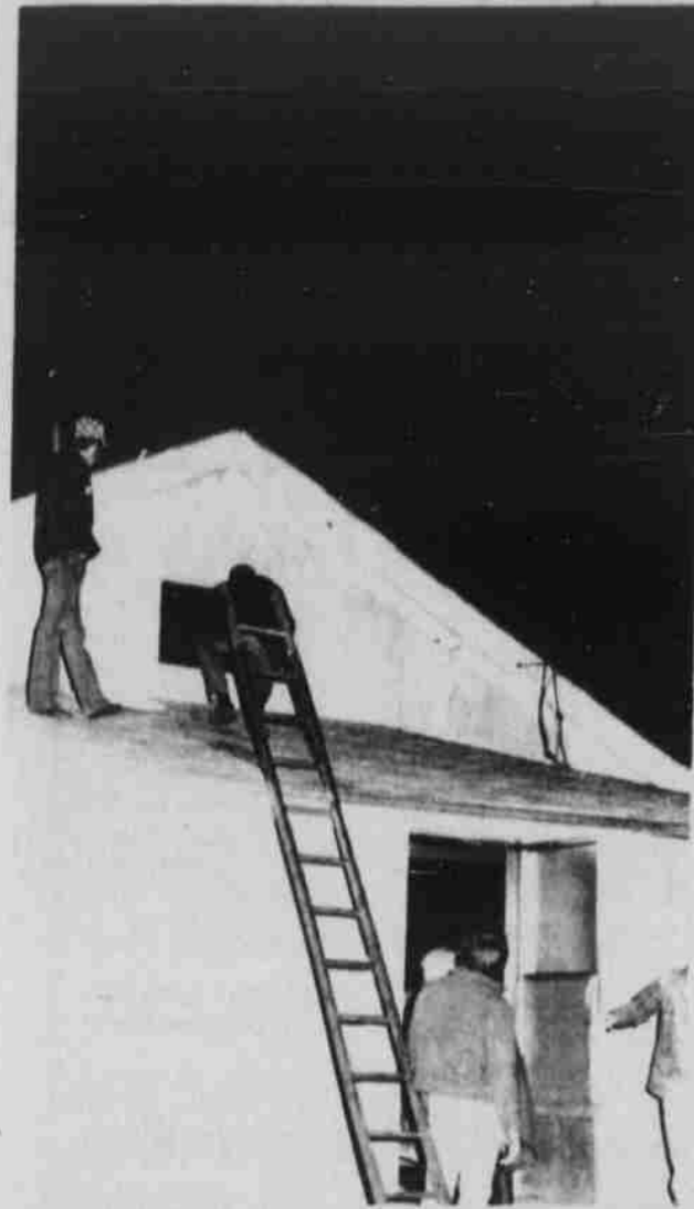
An alert Oregon State Police officer saw some smoke and thought someone was burning trash Saturday night. A closer inspection revealed the home of John Hanna smoldering. Heppner's volunteer firemen were called to the scene of the fire on Hinton Creek. The damage to the home is not known at this time. It is believed the fire started from a small electric heater that had been placed near some paper.
