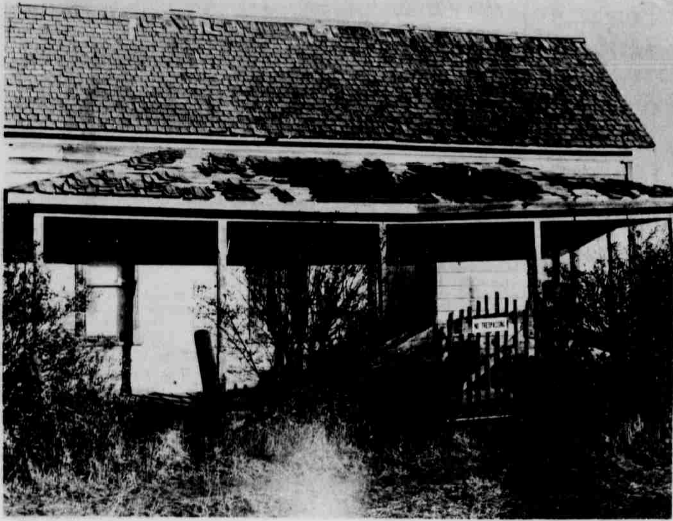
This charming old house at Hardman is typical of those in the ghost town area. The owner must believe a man's home is his castle, as witness the No Trespassing sign on the sagging gate.
