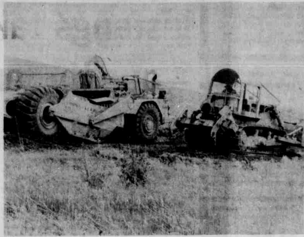
Valley View Estates owners lost no time getting men and equipment into action to lay out roads and streets for the new hillside residential subdivision above Pioneer Memorial Hospital.
