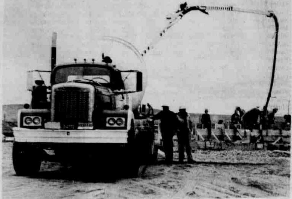
Workmen at Techbuilt Corporation are pouring concrete for the walls of its new building. When completed the concrete wall sections will be raised from their prone position and set into place. According to John Winget, superintendent for Techbuilt, work is proceeding ahead of schedule and the first section of walls should be in place by early May.
