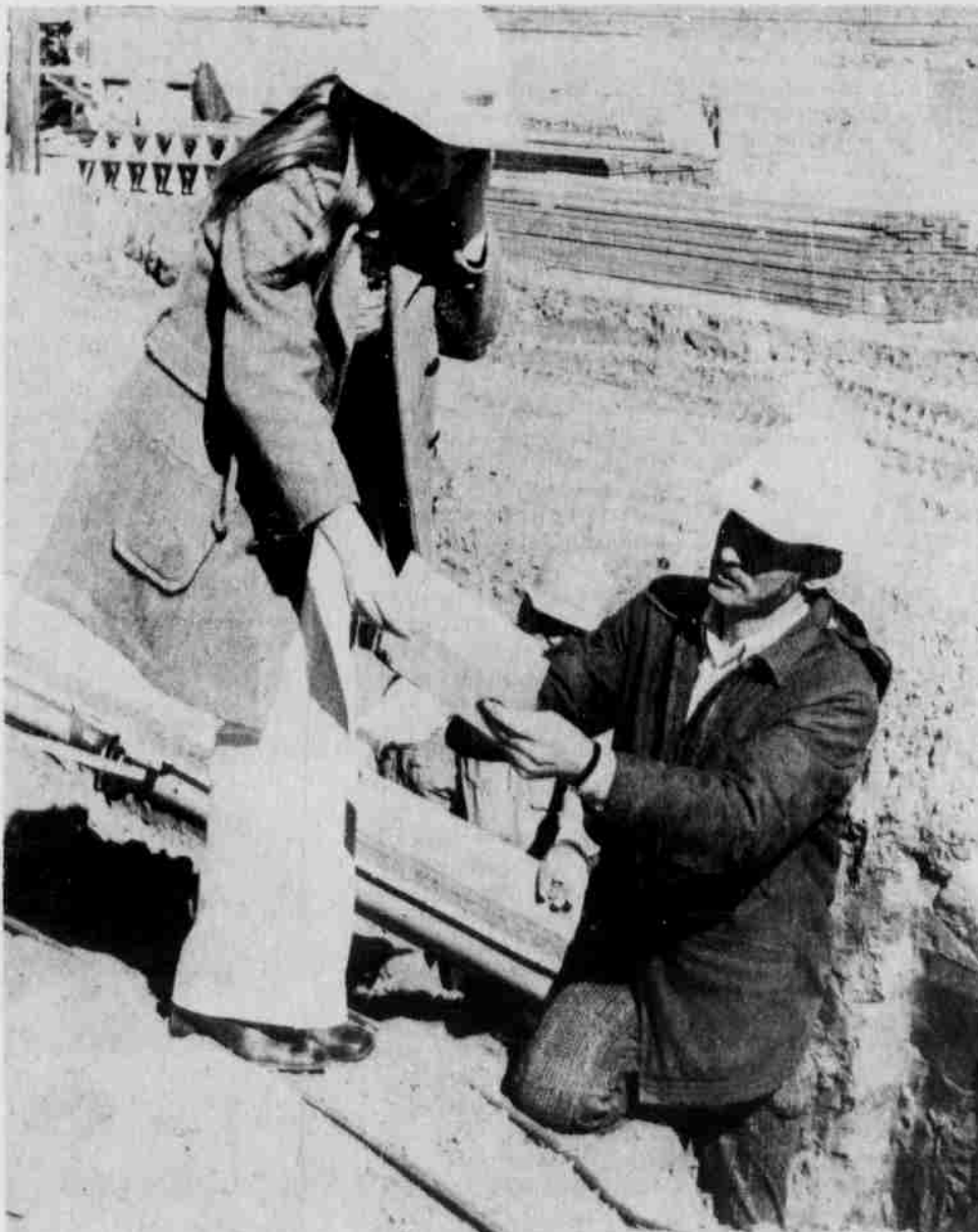
Lynell Braat, secretary for Techbuilt Corporation, interrupts Marvin Snyder, foreman, as the first concrete was poured Friday for the new Gourmet Foods complex near Boardman. Earth moving started three weeks ago. The building is to be completed by Aug. 1.
