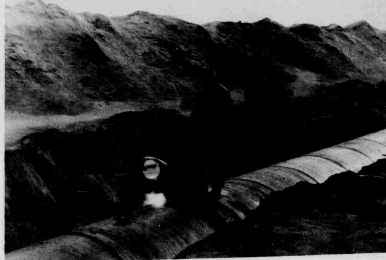
WATER TO THE DESERT —Employees of Sabre Corporation are shown welding links of the 72-inch irrigation main line on the property of Eastern Oregon Farms, south of Boardman. This is a part in the giant agricultural plan that will boost the economy of Morrow County.
