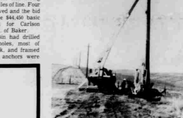
Pole setting is pictured here on the new Columbia Basin Electric 69 kv Ruggs Transmission Line. The new line will greatly improve service to the rural areas near Ruggs and Hardman.
