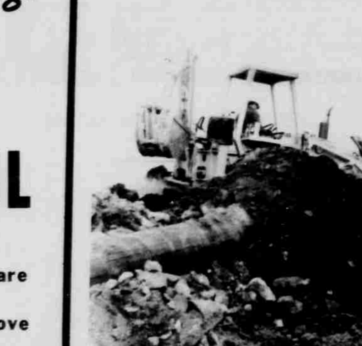
Pole setting is pictured here on the new Columbia Basin Electric 69 kv Ruggs Transmission Line. The new line will greatly improve service to the rural areas near Ruggs and Hardman.
