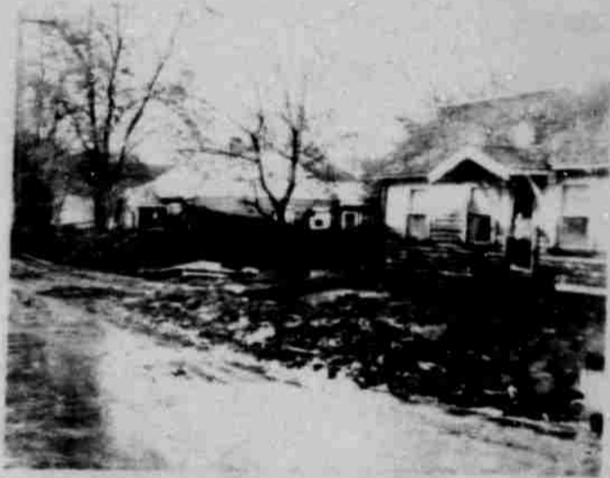
Serious damage by flood to Heppner homes.
