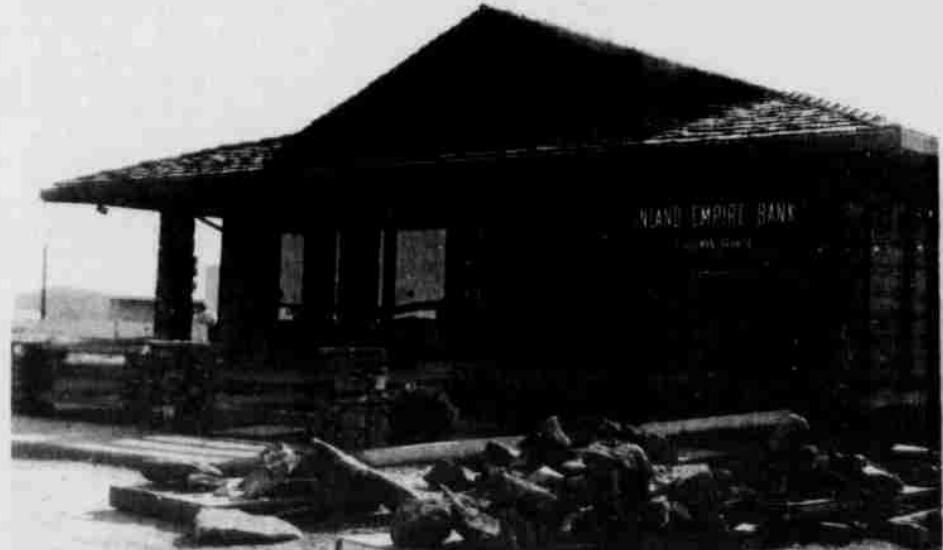
Inland Empire Bank at Boardman with its handsome stone and wood front. The rail fence in the process of construction encloses the landscaped area.
