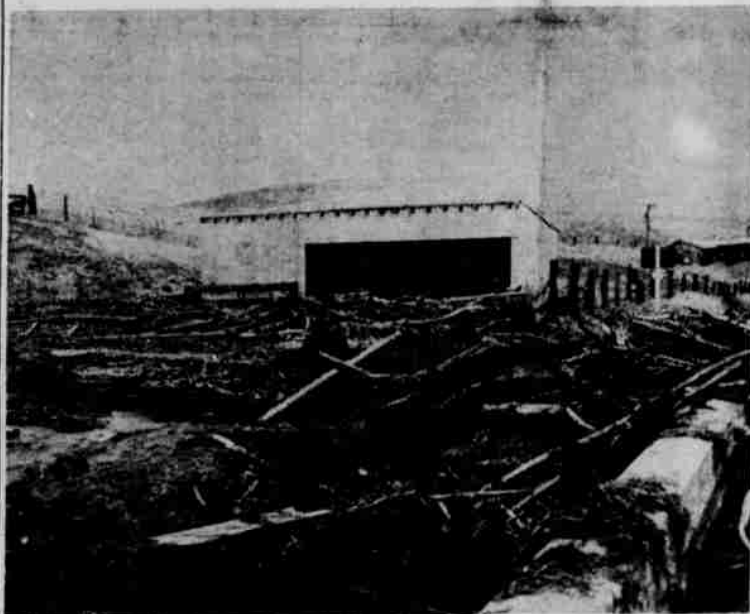
THIS PICTURE SHOWS Route 207 bridge in the lower right and Pettijohn's new barn in the upper center. The barn is about 10 feet higher than the bottom of the channel. The bridge has a 6 foot high opening and a 2.5 foot high railing. (SCS Photo).
