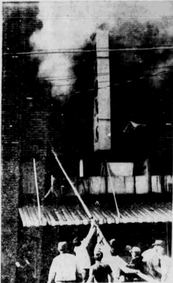
THE IONE PUMPER made the difference between this feeble stream of water with normal hydrant pressure as compared with the 100% increase when firemen put the lone Fire truck pumper on this line.
