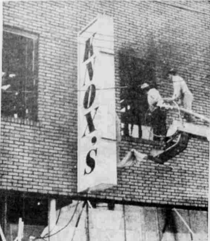
(FROM THE GAZETTE-TIMES, Nov. 11). The fire caught the roof and upper story of the Knox Dept. Store Building. Part of the Knox roof collapsed and much damage was done by smoke and water.
