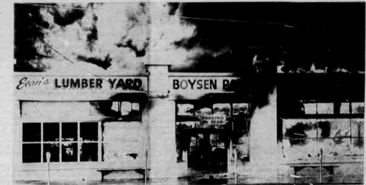
EVANS LUMBER YARD was all but gone when this photo was taken. The fire had already spread into the upper part of the Knox Building. Evans' entire roof had collapsed and shortly a large part of the Knox roof also collapsed. Loss of the two buildings and contents will run about $150,000. (G-T Photo)
