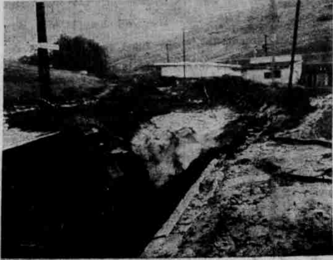
THE CHASE STREET bridge used to be here. Wall of water is shown receding. (Forest Service photo).
