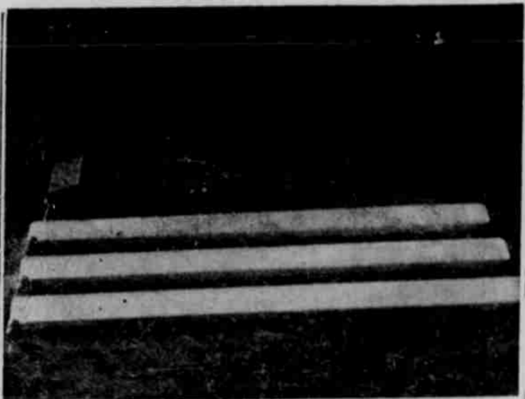
ALLEN TOM'S big chicken plant is shown here in a wheat field. Top left is the processing plant with the three laying plants below. Each of the large buildings houses 80,000 layers. Each building is the equal to one and one-half football fields.
