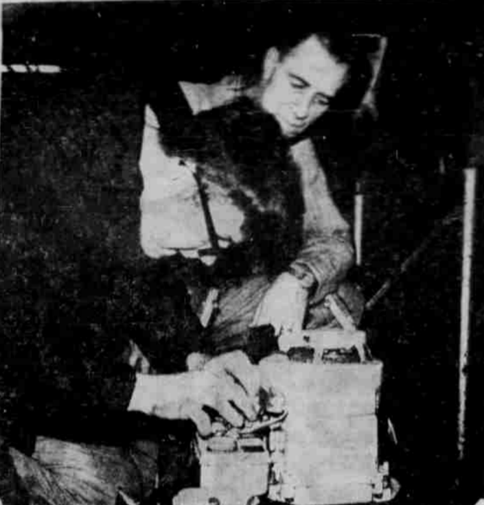
WORKING WITH small engines is another Riverside FFA study. However this is Doug Frichard, senior, Riverside FFA reporter, at a BMCC small engines class. He is working on a 2 1/2 HP lawn mower engine for his own use. Ron Black, Riverside FFA instructor stands ready to give an assist. Doug's favorite FFA projects are his Angus cattle.
