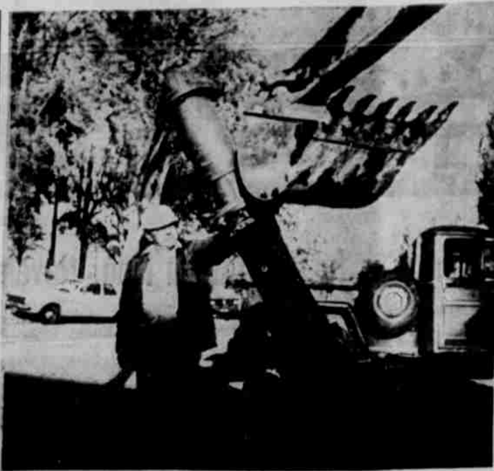
ELDON TUCKER prepares to lower the last Fire Hydrant to be installed in the current water improvement project at Ione.
