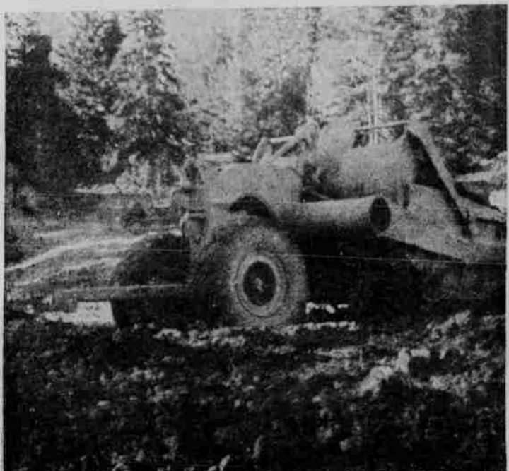
GETTING STARTED is a big earth mover that will haul many tons of earth and rock to form an earth-fill dam. At the tiller is Bill Weatherford. Mr. Light said he would guess that with weather permitting and no more break downs, they just might finish the main portion of the dam fill in about two weeks. The project is being built by the Lake Penland Corp., a group of private citizens, mostly from Morrow County, who are paying the bill. Harry O'Donnell is president of the corporation. The Oregon State Game Commission will stock the lake with trout. Group is receiving some engineering help through the Heppner Soil & Water Conservation District.
