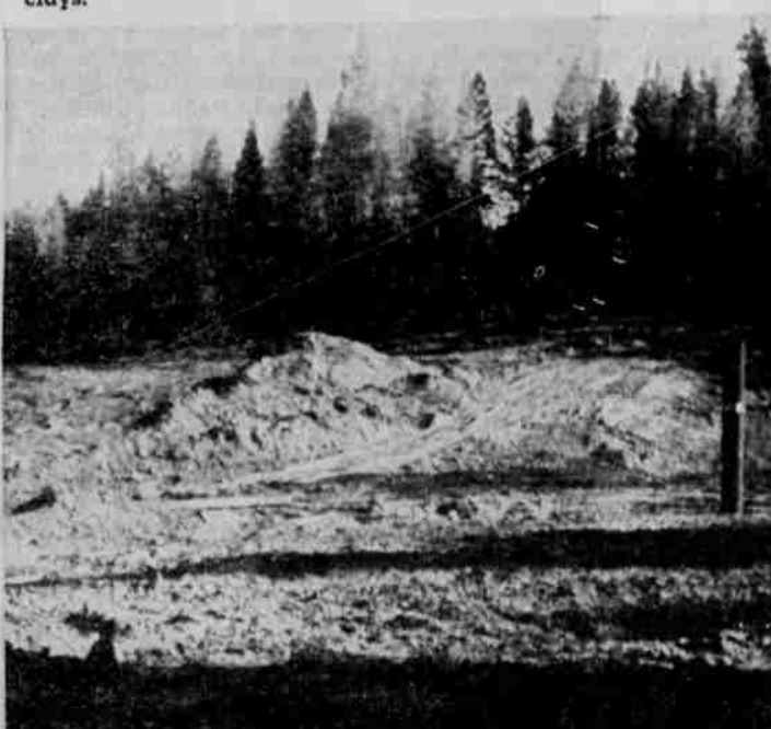
THE LAKE PENLAND project is nearly 50% completed. The concrete drain pipe is in and shown here is the upright standpipe. Top of the dam will be about 3 1/2 feet below the top of this pipe. Another larger pipe will cover the top of this stand pipe. A lateral pipe will lead into the upper part of the pipe to drain off acid water. The Oregon State Game Commission believes that freezing of the vegetation in a lake in the winter causes acid in the water injurious to fish. A drainage from the bottom near the dam will lead up near the top of the standpipe to drain off this acid water. Top of the dam will be about 350 feet long with a height of 139.4 feet high. Water elevation will be 136.4 feet.
