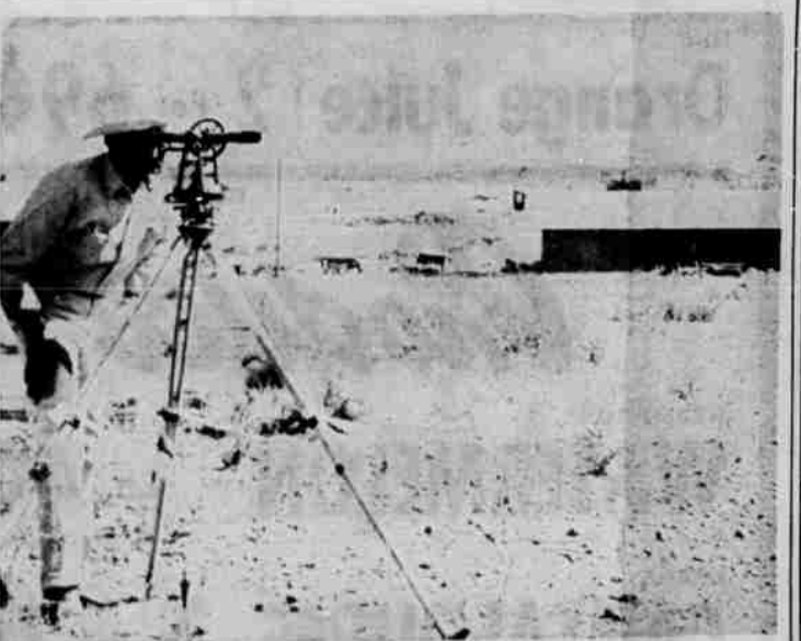
FIRST STEP in the construction of the new building at Kinzua. Dan McCluskey of Bend is on the transit to start laying out the building. Woody Ellison of Hermiston was assisting him. When fully completed, building at Heppner's Kinzua plant will house a plywood plant covering about 5 acres, employing 177 men.
