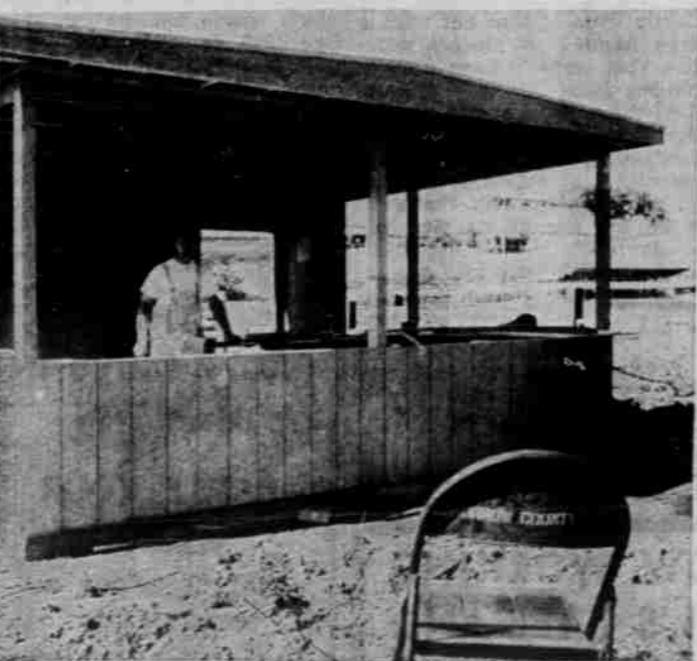
INSTANT SNACK SHACK . . . one day it was a slab of cement and three days later it looked like this. The lonely chair in the foreground is waiting for a happy hungry customer. Mel Piper is the carpenter.
